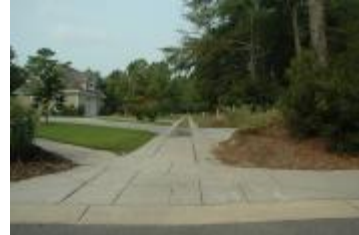
Example of alley paving
