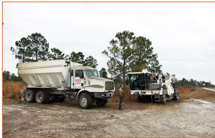
The contractor has begun to mobilize for the road repair project.
